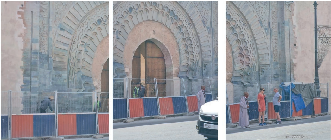
Figure 8. Bab Agnaou gate after the end of the renovation.
