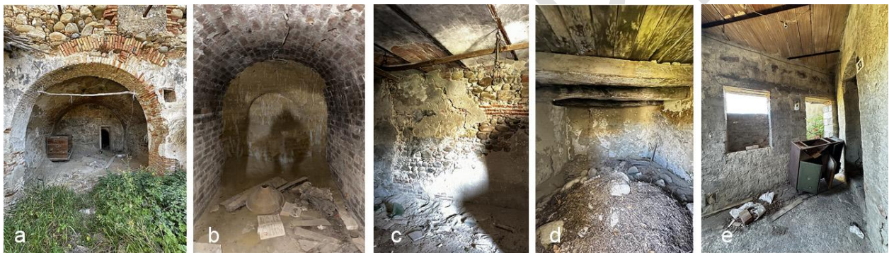
Figure 6 – a: brick barrel vault building 25b ground floor. b: brick barrel vault building 25a cellar ground floor. c: floor with beams and vaults (beams with deformable slab) building 25a ground floor. d: wooden floor with simple framework planking (beams with deformable slab) building 25d ground floor. e: floor with beams and large planks (beams with semi-rigid slab) building 25a first floor. © 2024, Authors.
