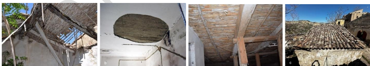
Figure 7 – a: roofing of building 25b beams, reeds, and tiles. b: roofing of building 25a, 2nd floor room under expansion. c: roofing of building 25a beams, reeds, and tiles. © 2024, Authors.
