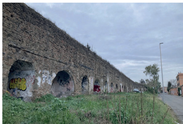
Figure 1. The Acqua Felice aqueduct. Source: The images were taken by the author during fieldwork.
