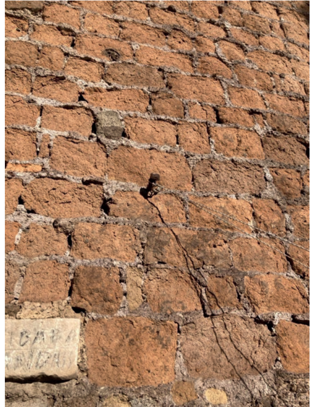
Figure 7. Close-up of the anchoring point. Source: The images were taken by the author during fieldwork.
