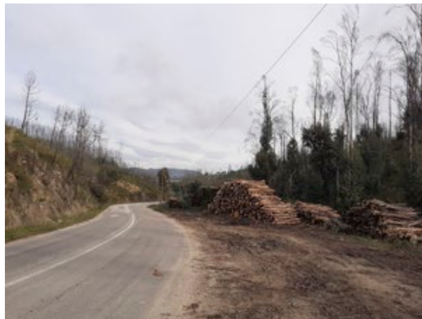
Fig. 2. The road from Lousã to Serpins that crosses a baldios area in October 2019. It was burnt by the wildfires of October 15 th , 2017. Dead pines are still standing, but Eucalyptus and Acacia species are resprouting to form a 'zombie forest', accumulating fuel until the next fire event. The wood trade operates at the sight of all without the legal permission of the commoners.
