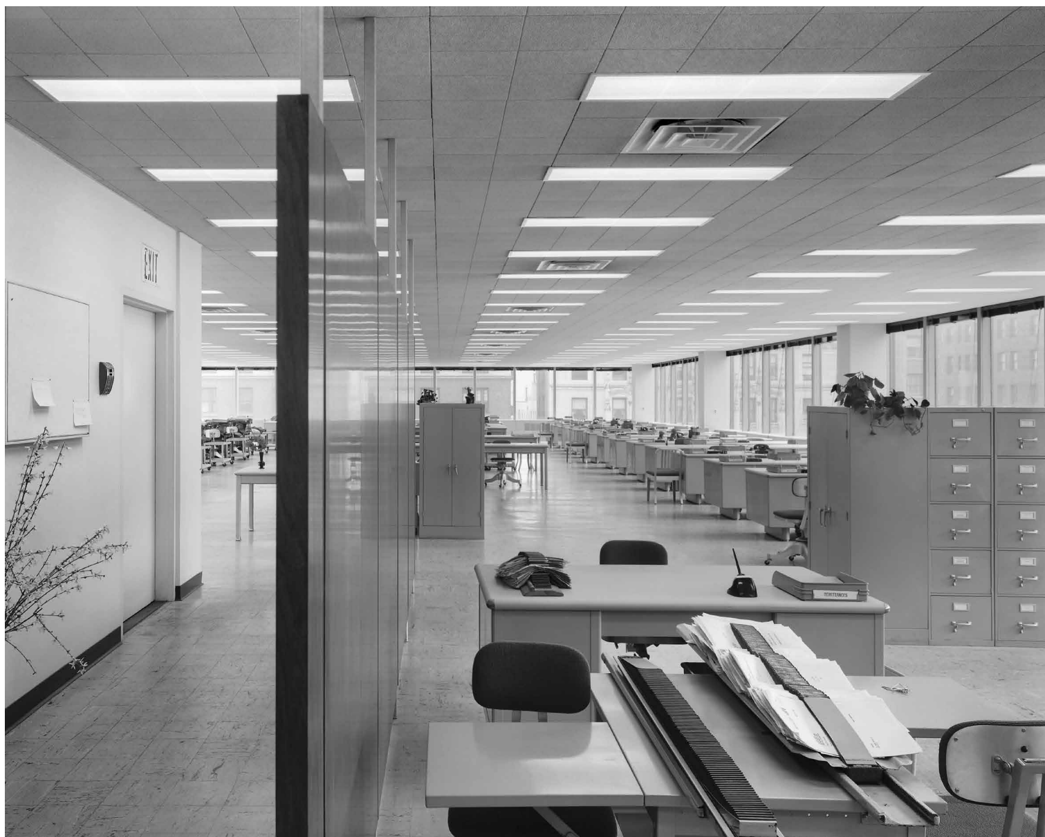
Fig. 8 Skidmore, Owings, and Merrill (architects); G. Bunshaft (chief designer); Jaros, Baum, and Bolles (mechanical engineers); R. Loewy (interior designer), Lever House, New York City, 1950-1952. Office interior, showing central air diffusers in the acoustic ceiling (© Ezra Stoller/Esto).
