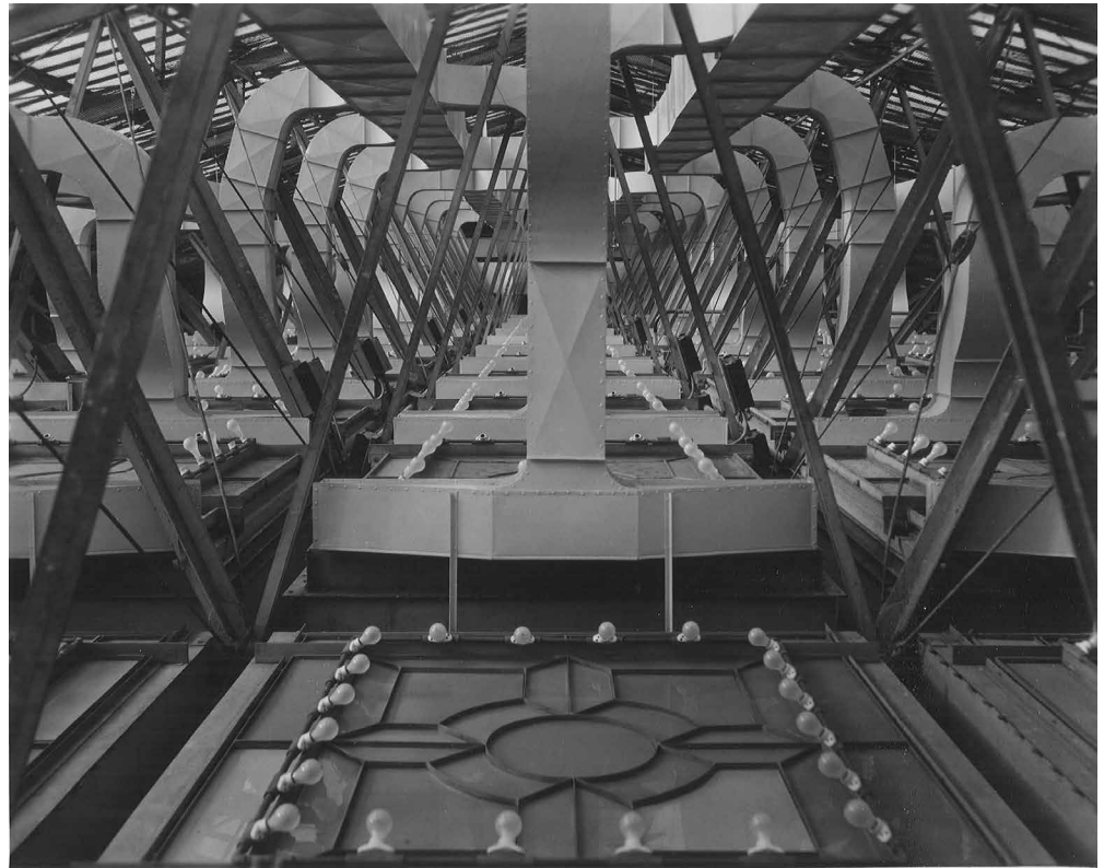
Fig. 7 U.S. Capitol, House of Representatives, Washington, D.C. Attic viewed along its center line, showing air conditioning ducts (installed in 1928) between iron trusses (installed in 1857), with diffusers along the base of the ducts at the edges of glass ceiling panels (from “Heating, Piping, and Air Conditioning”, 1, 1929, 8, p. 66; © Carrier Corporation Archives, Iron Mountain).
