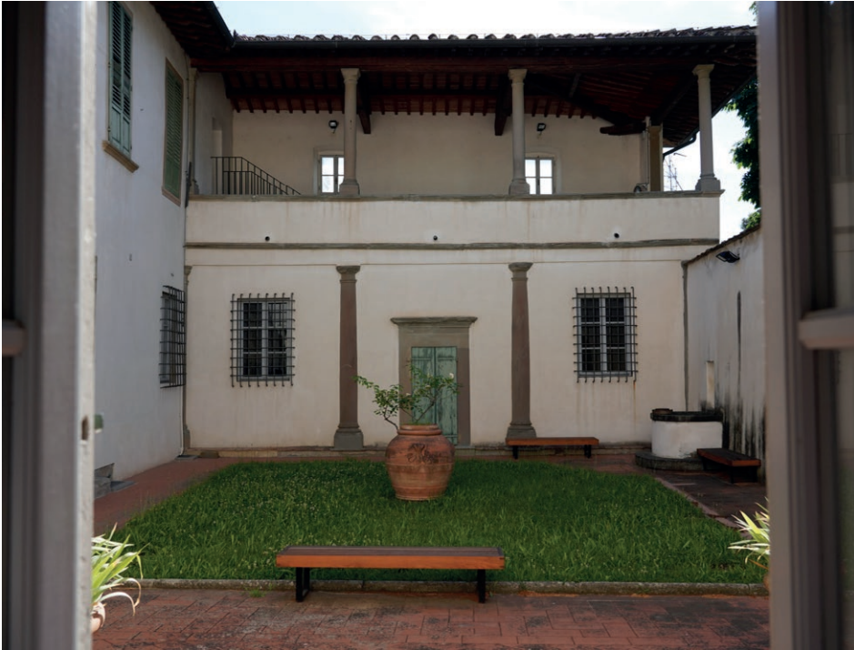
Figura 2. Il cortile della Villa e l'altana, come appaiono dopo il restauro terminato nei primi anni del 2000. Figure 2. The courtyard of the Villa and the roof terrace, as they appear following restoration work completed in the early 2000s.
