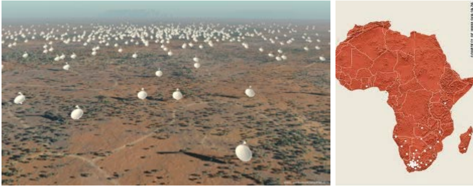
Figure 1. Left Panel: an artist's view of the core of the Mid Array antenna complex. The streets portrayed give an idea of the overall dimensions. Each antenna will have an offset Gregorian design with a height of 15 metres and a width of 12 metres. Right panel: a proposed large-scale antenna distribution in Africa.
