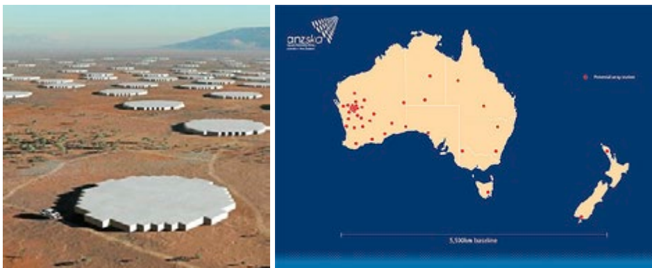
Figure 2. Left Panel: an artist's view of the core of the Mid Array antenna complex. The car portrayed gives an idea of the overall dimensions. Each white enclosure comprises 256 small antennas. Right panel: a proposed large-scale antenna distribution in Australia. The New Zealand locations will probably be dropped.
