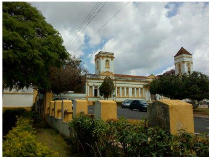
Fig. 19 – The old railway station in Araxá, converted into a cultural centre. Courtesy of the Author
