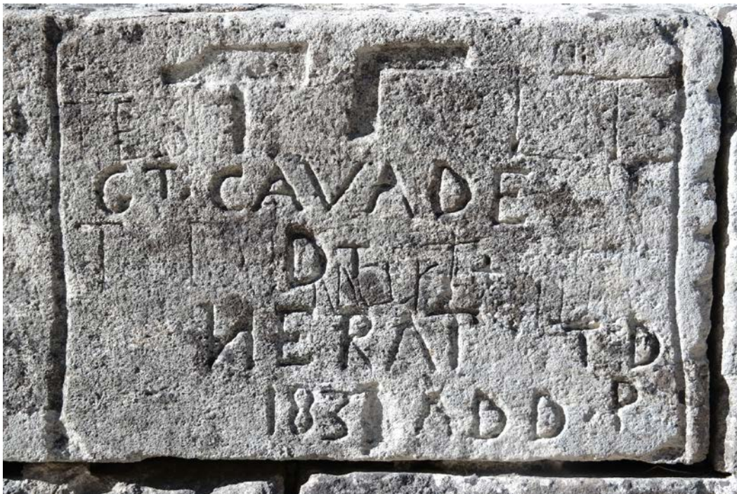
Figure 6 – Graffito at Pont du Gard (1831). Photo by Polly Lohmann. Courtesy of the Author
